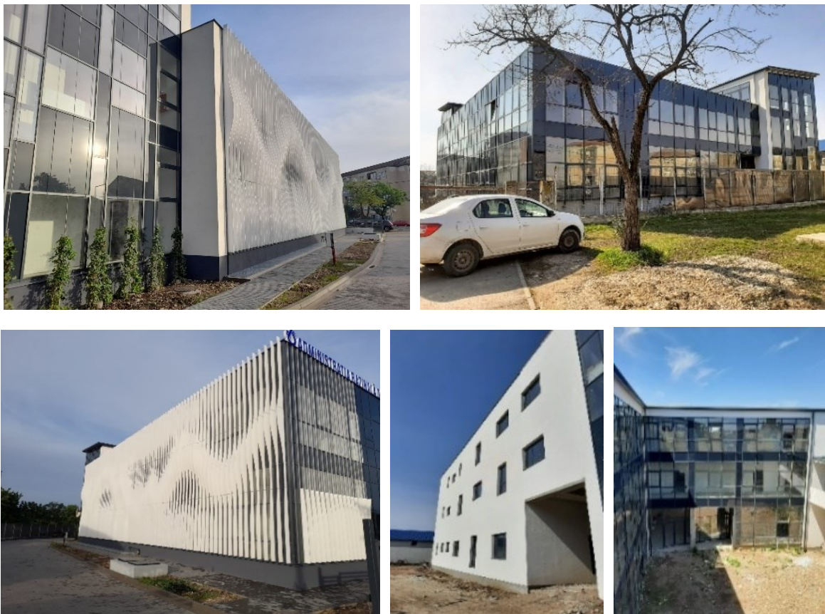
Figure 2.4.2 Left side photos 26.06.2023, Corian material vertical waved sunshades mounted partially/ Right side photos 27.05.2021, execution stage.
